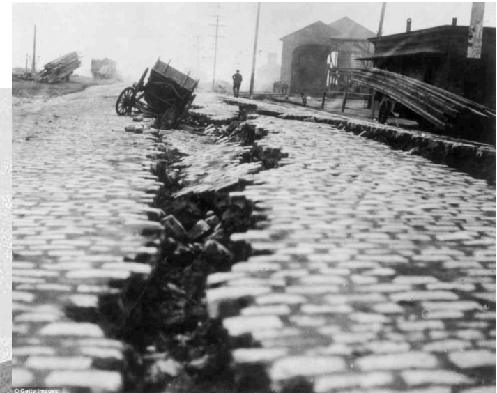
A cobblestone street, which was split down the middle after the Great Earthquake in San Francisco, California, in 1906
