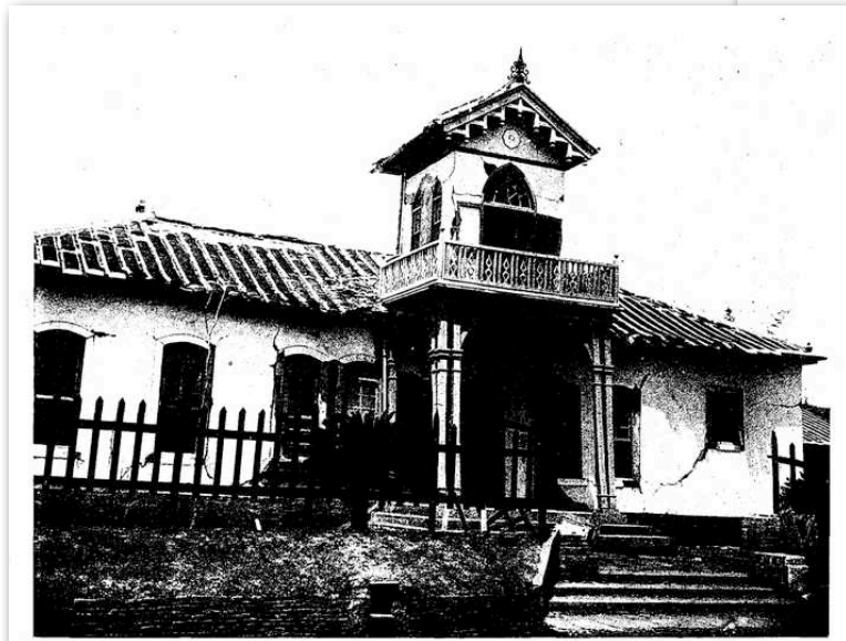
Fig. 8. The New Sub-Prefectural Office Shinko, showing the effects of vibration of the front tower. The building was of wood, with plastered walls.
