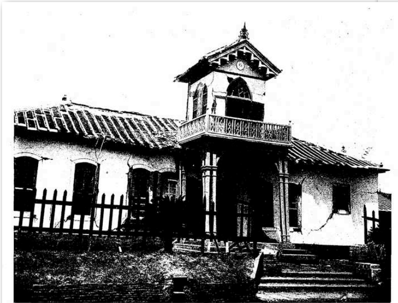
Fig. 8. The New Sub-Prefectural Office Shinko, showing the effects of vibration of the front tower. The building was of wood, with plastered walls.
