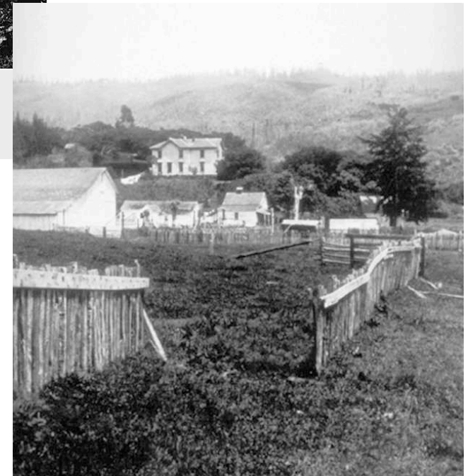
Near Bolinas in Marin County. Picture by G.K. Gilbert showing a fence that was offset about 8.5 feet along the trace of the fault (from Steinbrugge Collection of the UC Berkeley Earthquake Engineering Research Center)
