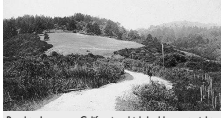
Road to Inverness, California, which had been straight before the earthquake of April 18, 1906, offset twenty-one feet where it was crossed by the earthquake fault. - H.O.W., California Earthquake Investigation Commission. (J. B. Macelwane Archives, Saint Louis University)
